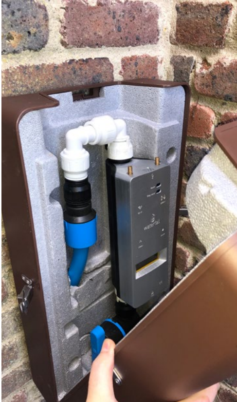
Figure 1 The Waterfall device fits neatly into the insulated, surface-mounted Groundbreaker system.
